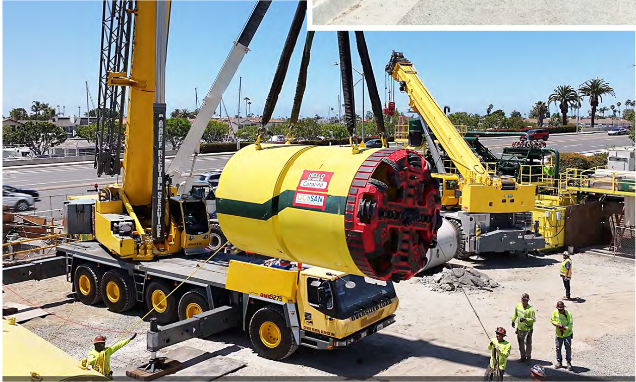
Crews work to lower the microtunneling machine into the launching pit
