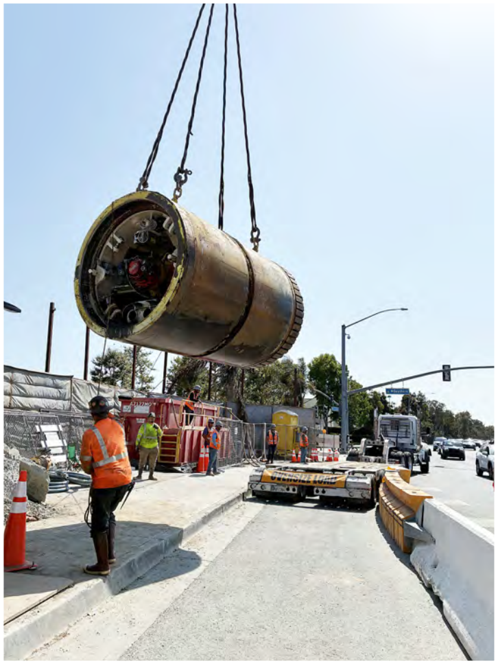
Microtunneling machine has completed tunneling and put onto a truck
