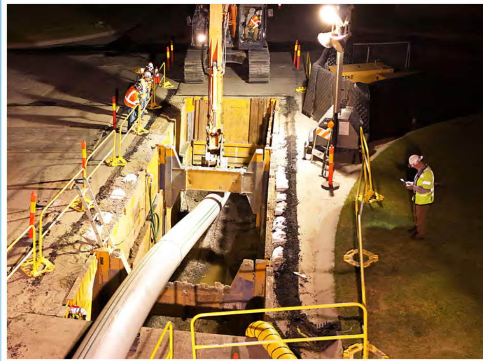
Pipe bursting, a construction method used to upsize pipes
