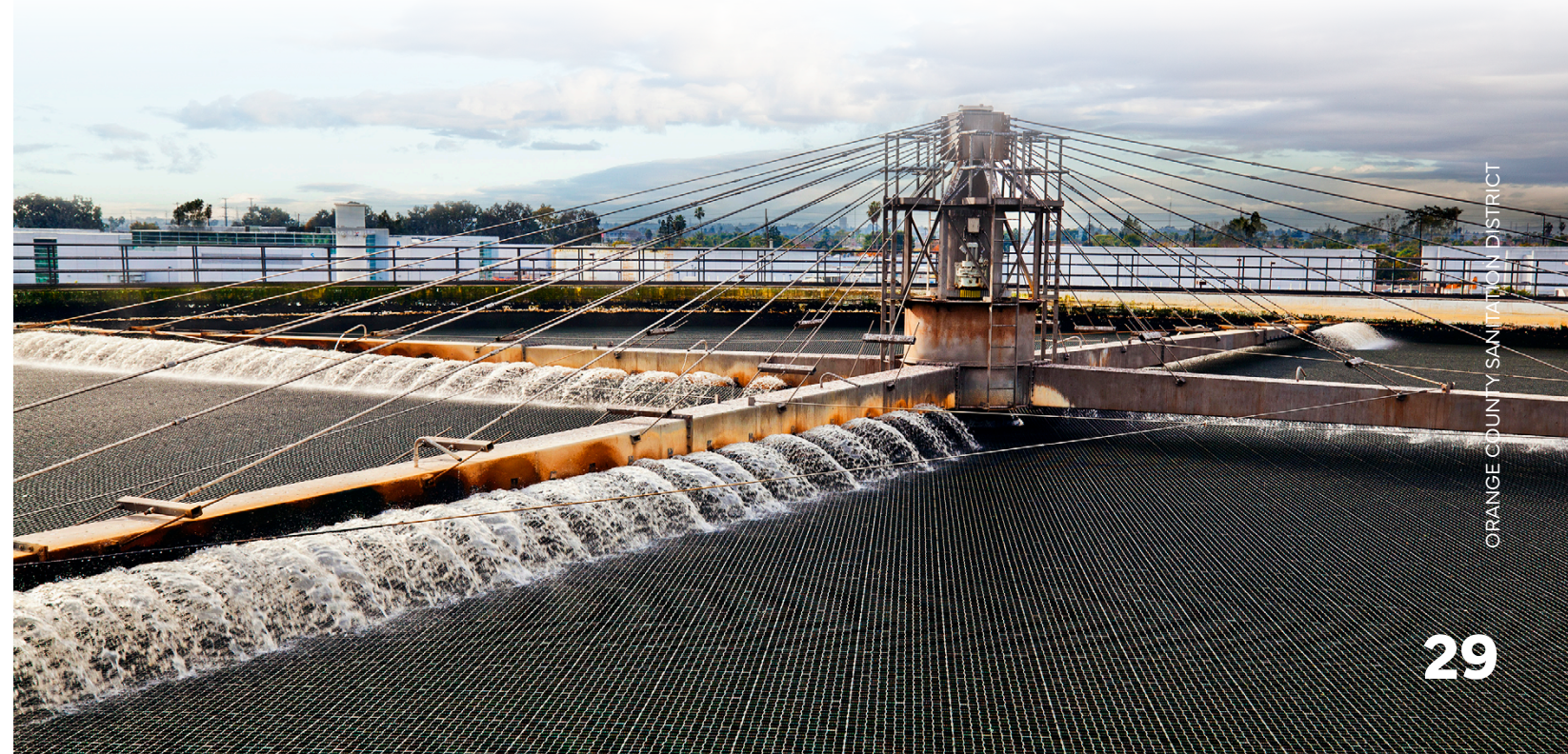
Construction of trickling filters.
