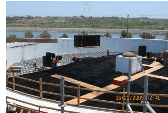
Construction of trickling filters.
