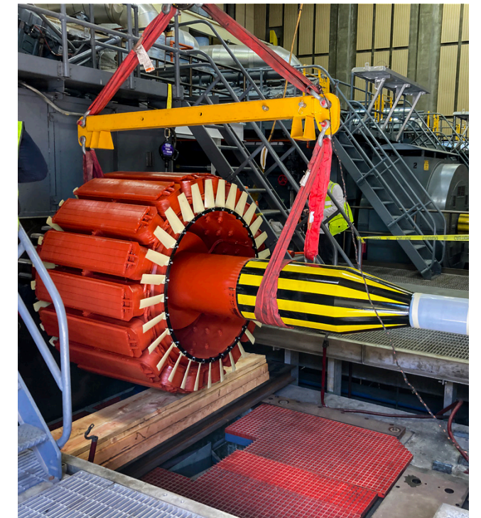
Overhaul of the engines and generators at Plant No. 2.
