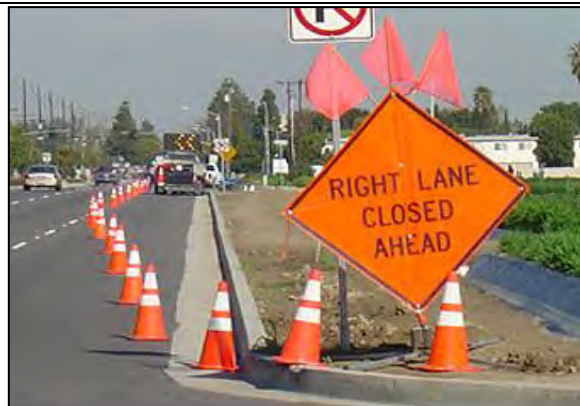
Figure 1: Traffic Control, Lane Closure (typical)
