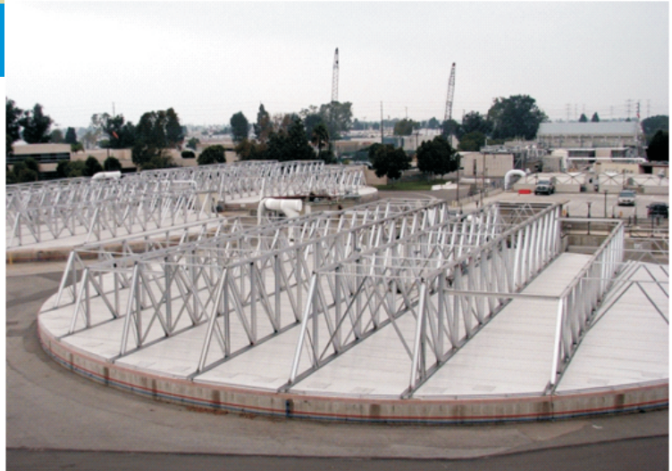
Primary clarifiers at Plant No. 1 with recently replaced flat covers.
