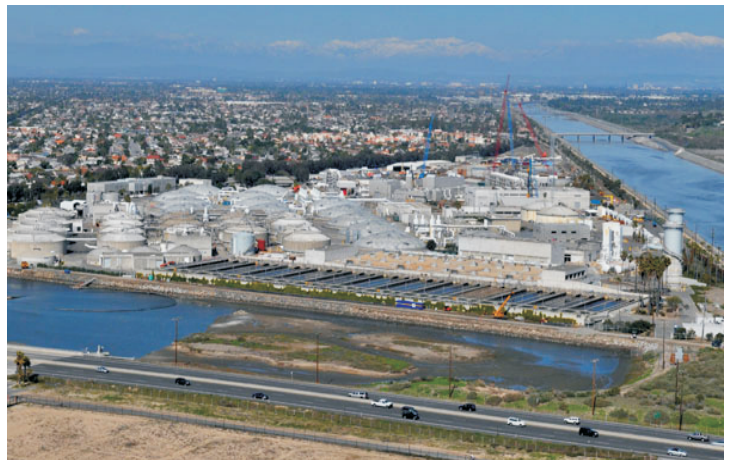
Treatment Plant No. 2 in Huntington Beach 2009.
