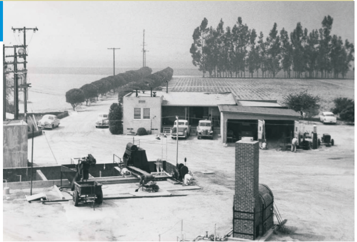
Treatment Plant No. 1 in Fountain Valley 1955.
