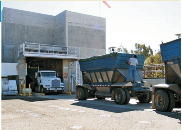
About 130,000 wet pounds of biosolids are produced each day.
