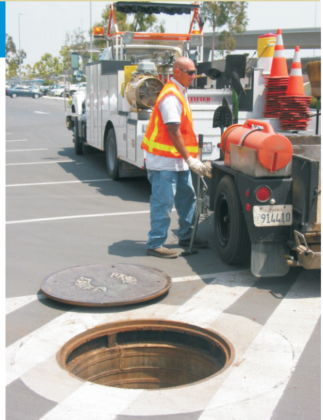
Collection crew cleaning a sewer line.
