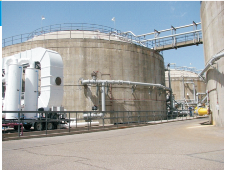
Solids removed from both primary and secondary treatment are sent to digesters.
