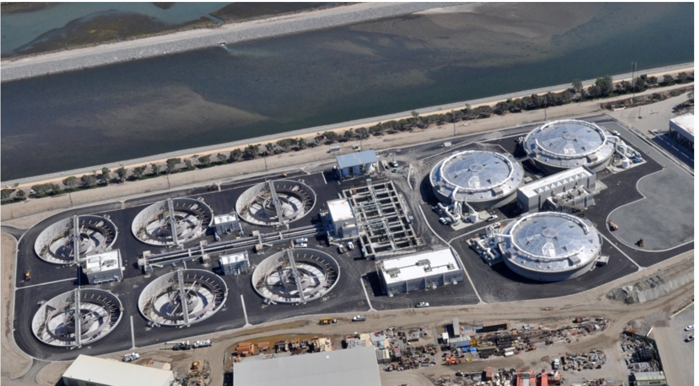
The construction of Trickling Filters at Treatment Plant No. 2 was completed in December 2010, two months ahead of the EPA consent decree milestone due date.
