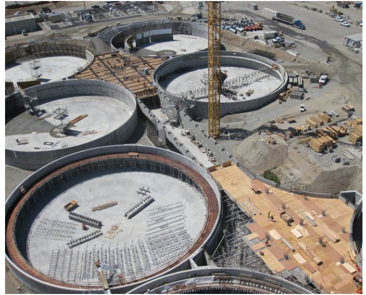
New secondary treatment system facilities in construction at Plant No. 1.
