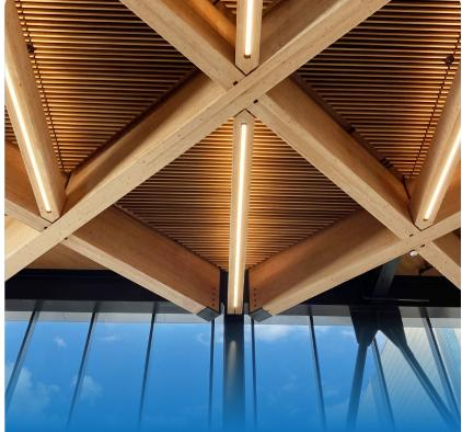
The building design integrated the most environmentally friendly features and materials including a hybrid of mass timber columns and decking combined with exposed steel-braced framing.
