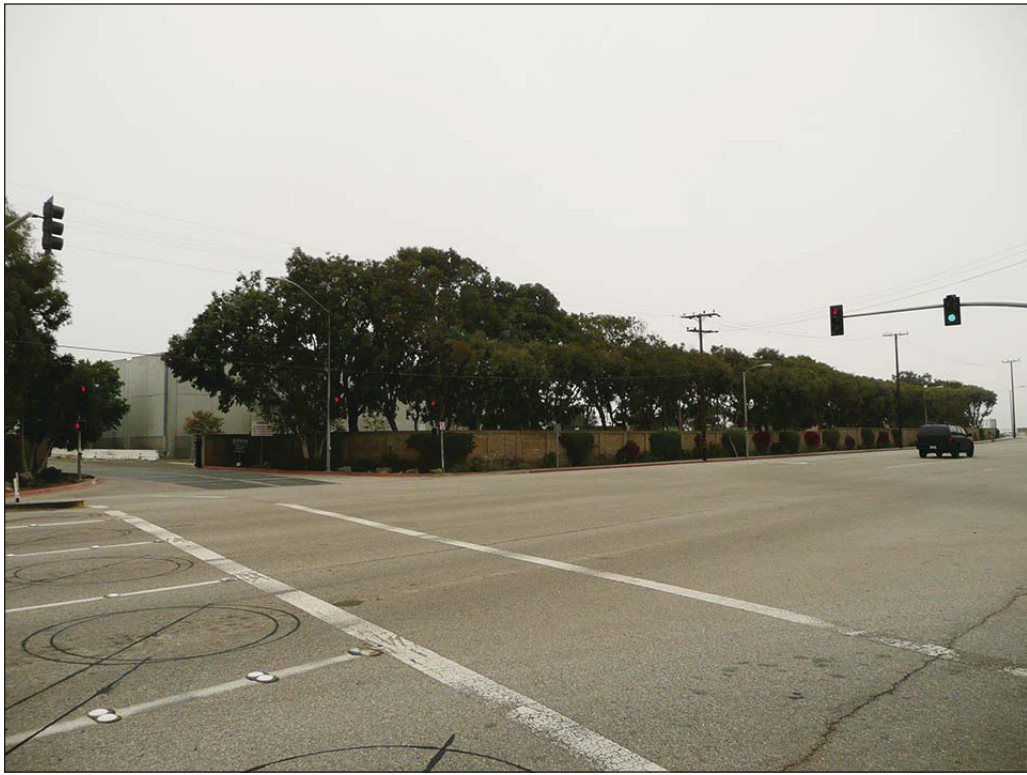
Viewpoint 1: Existing view of Plant No. 2 from Brookhurst St. and Bushard St. intersection looking southeast
