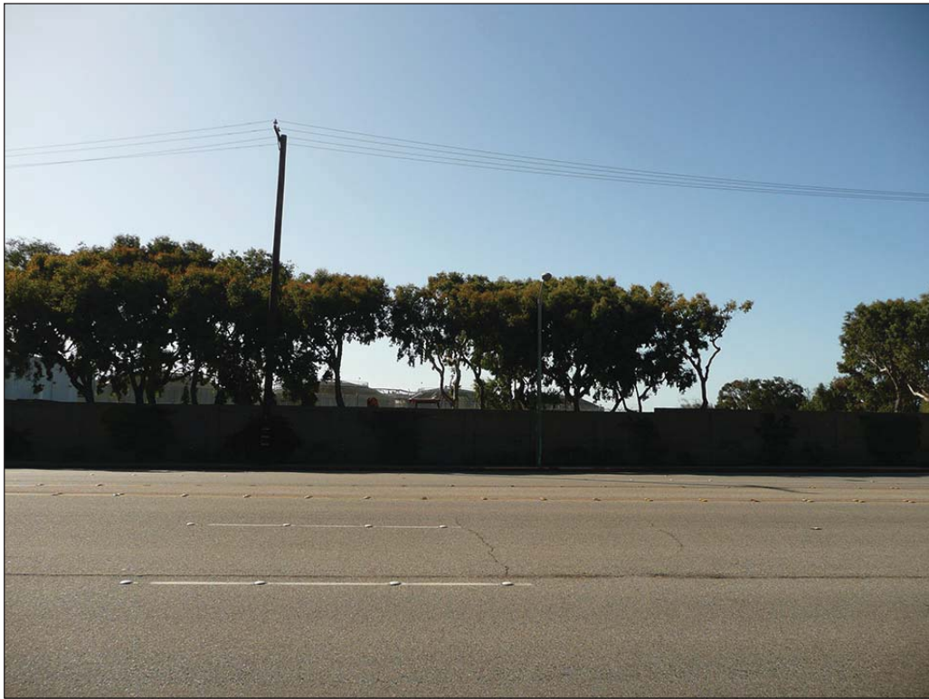
Viewpoint 2: Existing view of Plant No. 2 from Brookhurst St. looking east
