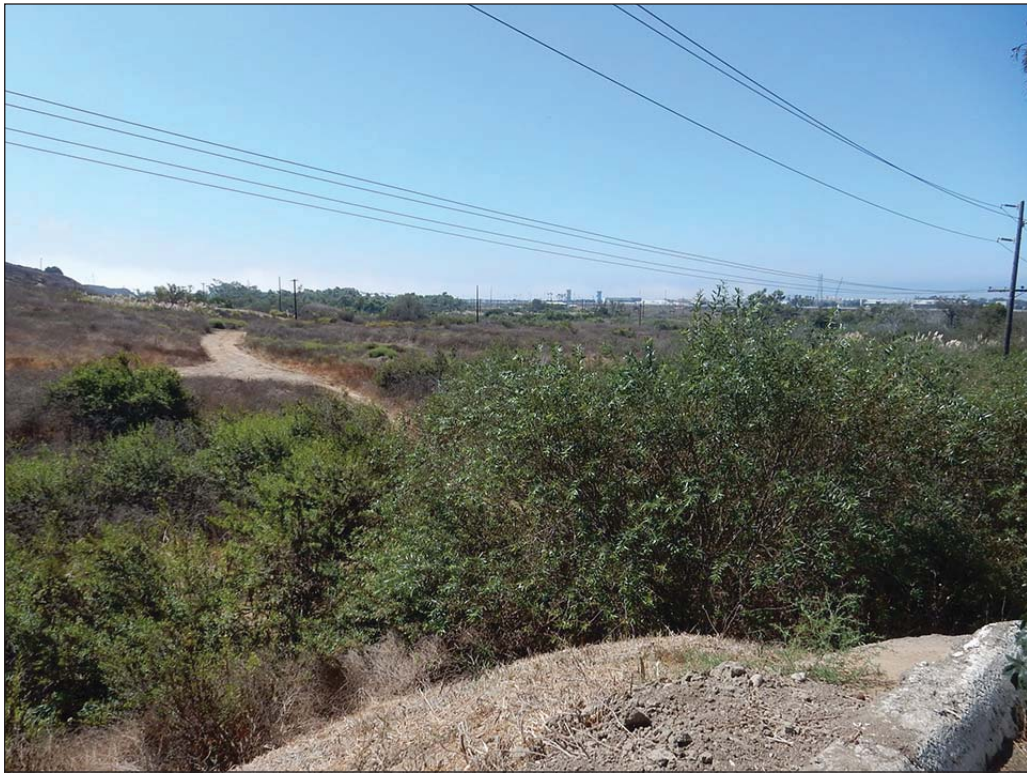
Viewpoint 9: View of Plant No. 2 from 19th St. and Balboa Blvd in Costa Mesa looking southwest
