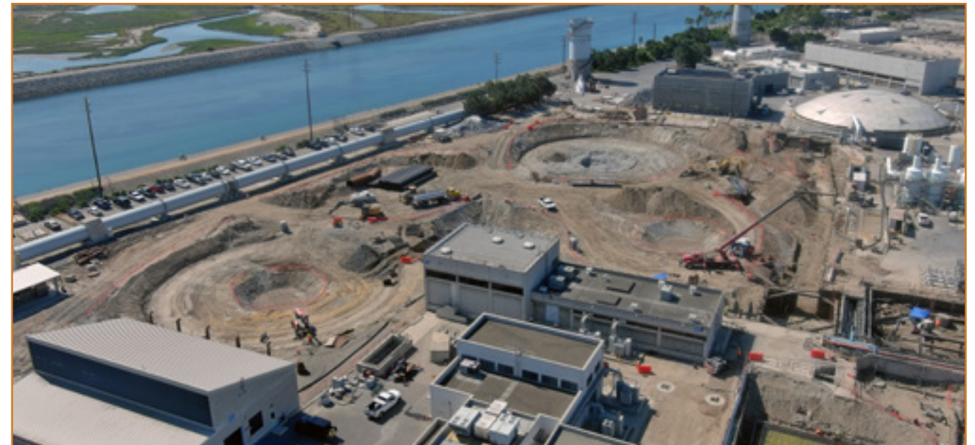
A-Side Primary Clarifiers Replacement at Plant 2 in Huntington Beach.
