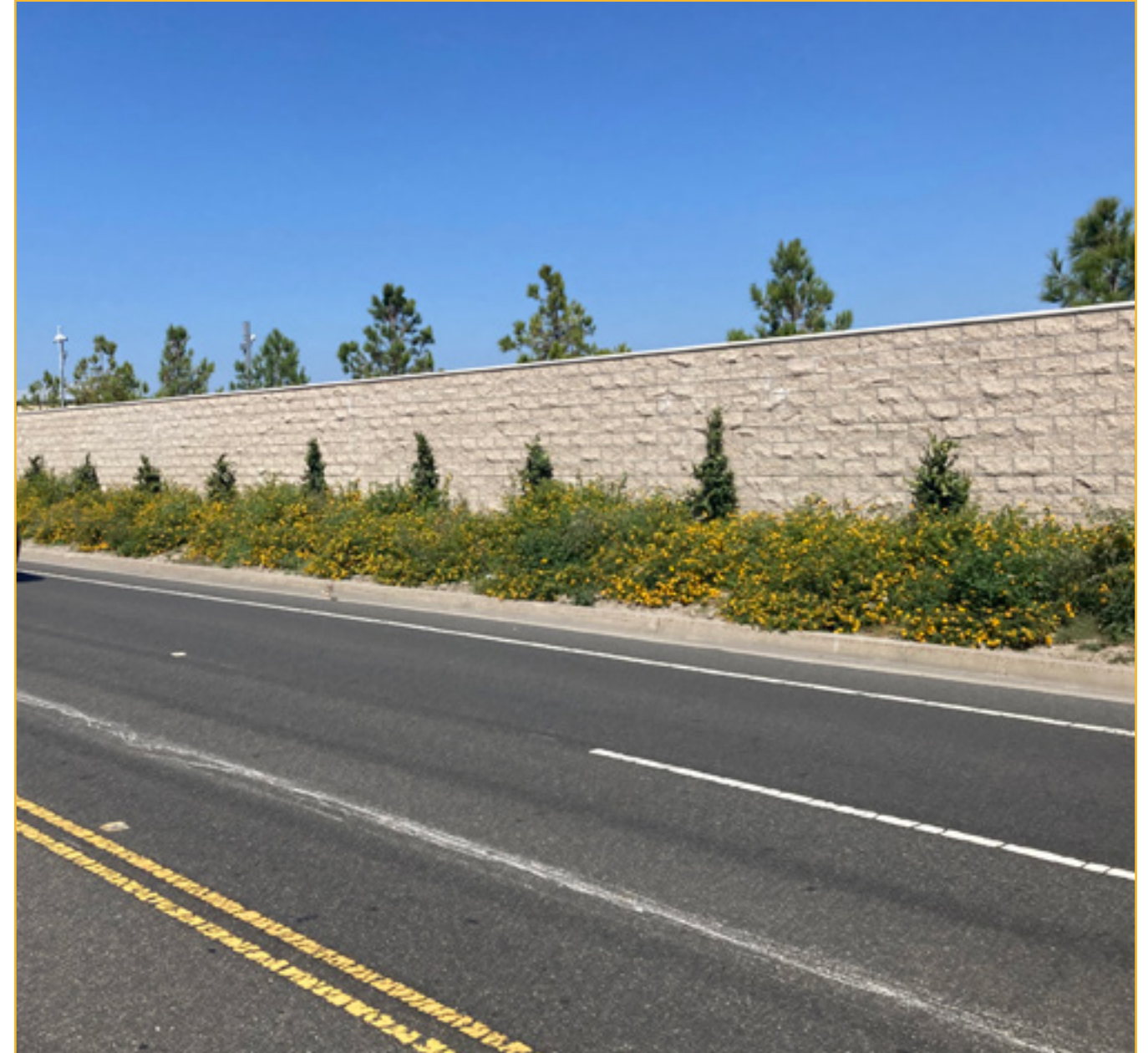
Street view of the new wall and landscaping for the Southern Perimeter Security and Utility Improvements Project.
