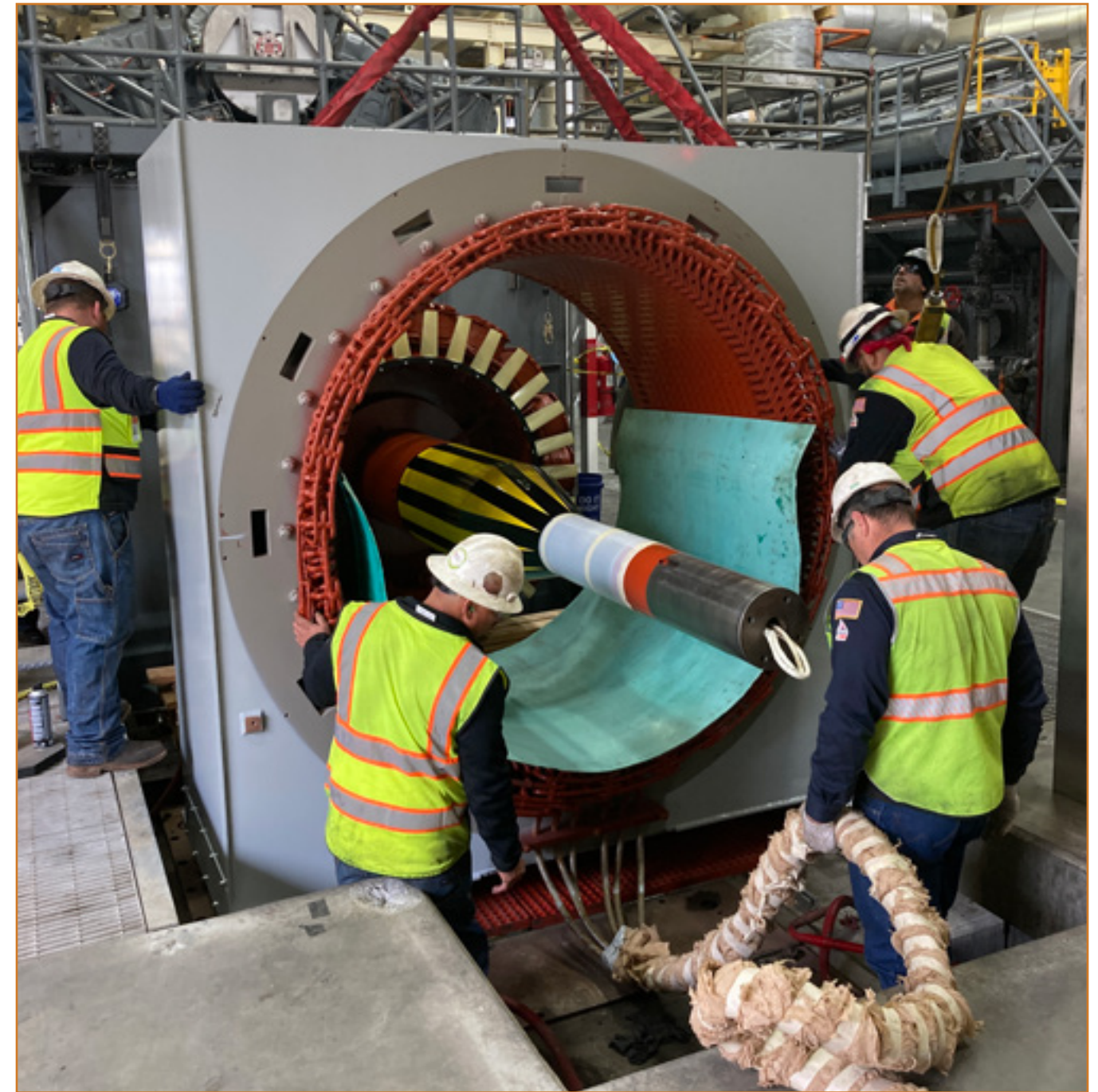
Engine and Generator Overhaul Project at Plant No. 1.
