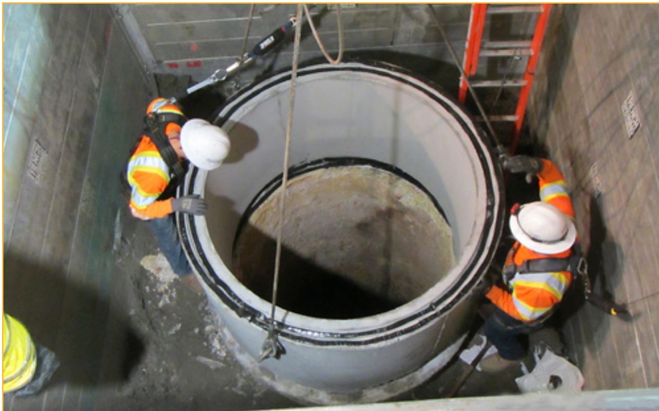
Manhole work on the Los Alamitos Trunk Sewer Rehabilitation Project.
