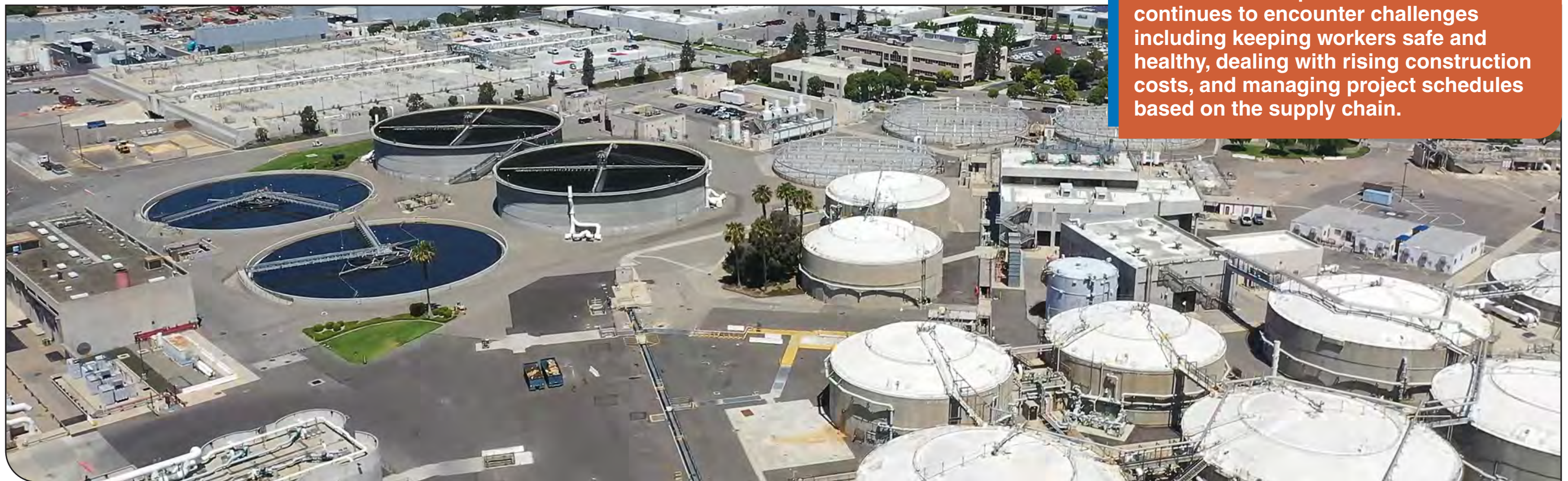
Reclamation Plant No. 1 in Fountain Valley.
