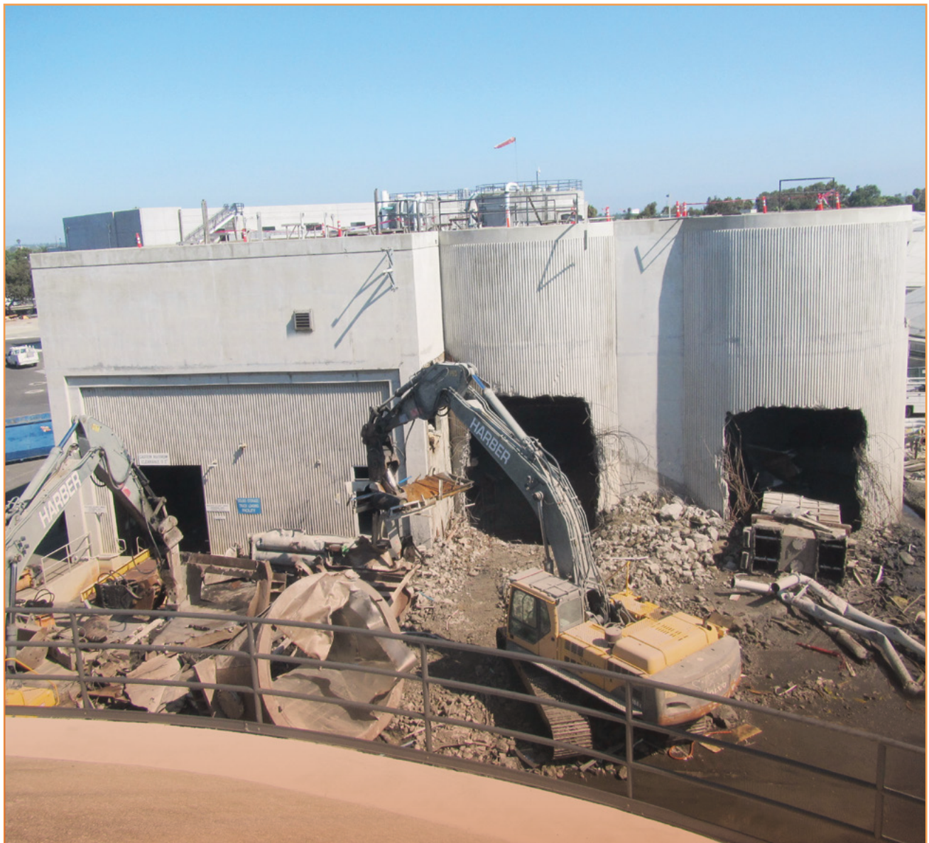
Demolition of the old truck loading bays at Plant No. 2.
