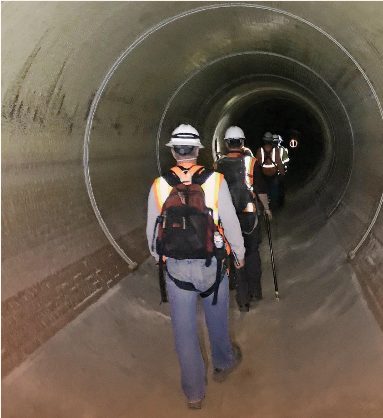
Walk-through inspection of the 120-inch pipeline for the Interplant Effluent Pipeline Rehabilitation project.
