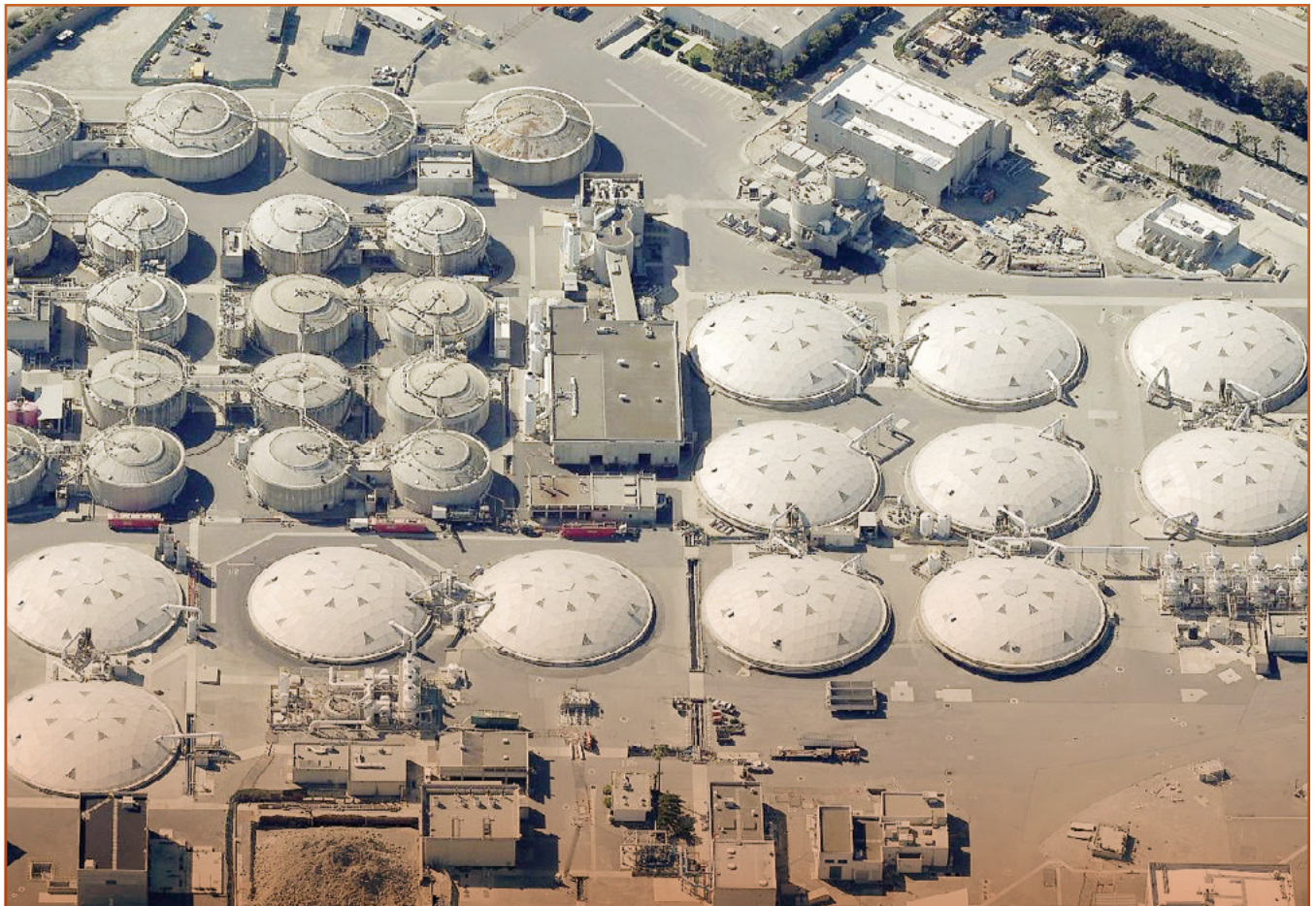
Aerial view of Plant No. 2. The larger circular geodesic domes are the 14 Primary Clarifiers.
