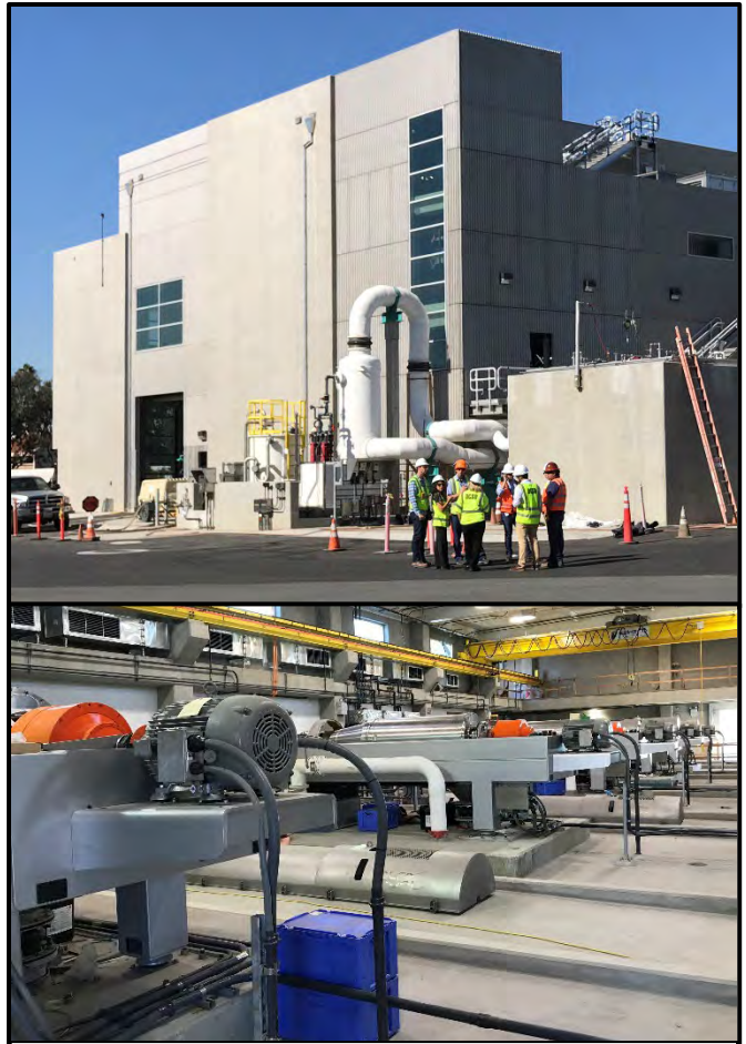
P2-92 Building and Centrifuges
