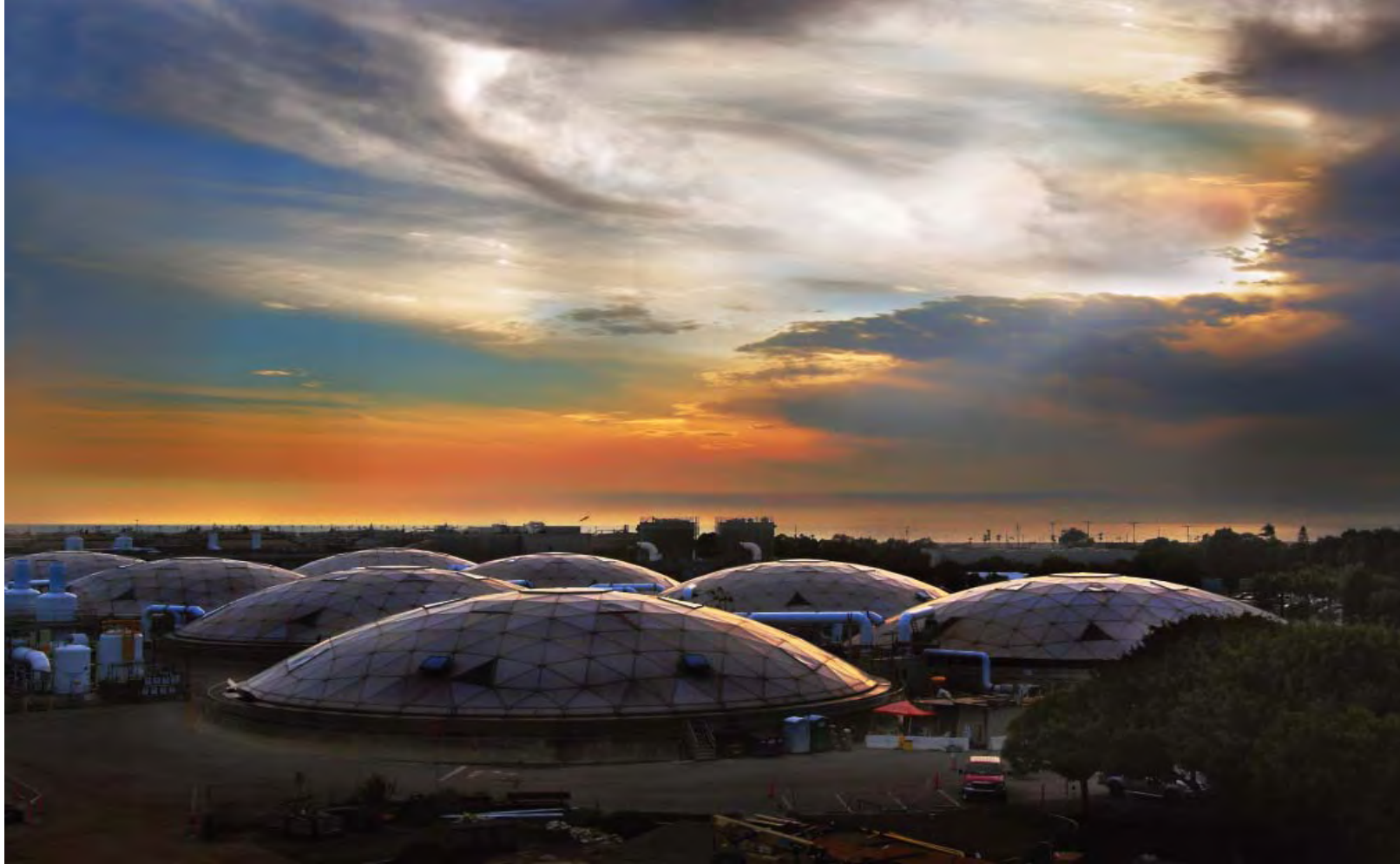
Operator Ddaze Phuong won the first prize photography award from the California Water Environment Association this year for this photo he took of OCSD Plant No. 2 primary clarifier basins at sunset.
